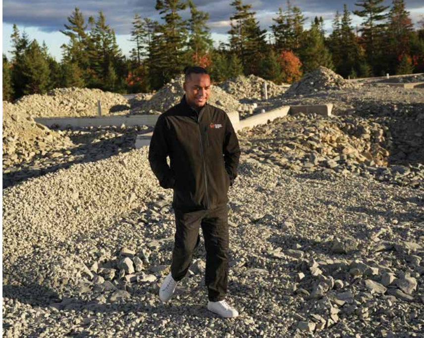
David stands on the site where 136 co-operative units are set to be built in Upper Hammonds Plains, Nova Scotia
