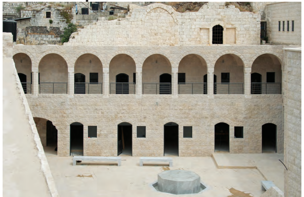
BELOW: The Khan al-Wakalah was built in the early 17th century out of local Nablus stone. After its restoration, Elias Khuri and Davide Pagliarini were brought on to design the courtyard, paving and new openings; they used readily available Carrara marble for the public furniture.
